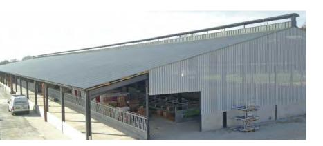
HIGHLIGHT is a perforated steel side cladding sheet that gives superb ventilation combined with natural light transmission.
